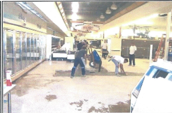
Concrete Placed In Trenches
