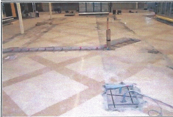
Trenches Ready For Concrete
